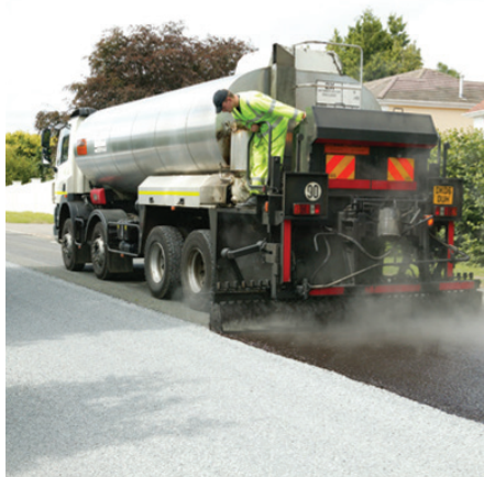
Bitumenemulsion, ytbehandling.
