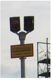
There are red light signals at some of the roads leading to the process area. When these are activated (red signal), the process area is sealed off and the signal must not be passed in the direction of the CKR/process area (see image).
