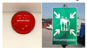
In office buildings, laboratories and certain other buildings, smoke, gas and high temperature detectors are installed. In case of fire or smoke development, the detectors will be triggered and emit a local alarm of fire bells and send an alarm to the Refinery rescue Services.
