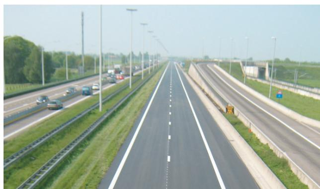
Phase two involved the resurfacing of 8km of the E19 between Loenhout and Brecht. Approximately 20,000t were removed over four days; 14,000t of asphalt base layer were manufactured and laid over four days and 6000t of surface course containing the PMB were laid over two consecutive days. Road markings were applied and signing removed.
