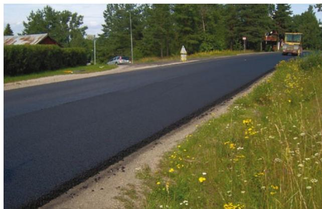
The concept can also be used for highly trafficked roads in place of conventional hot mix asphalt. The lower production temperature reduces over time ageing of the bitumen, which increases the lifespan of a pavement. With foamed bitumen, it is also possible to use large amounts of recycled material without reducing the quality of the product.
