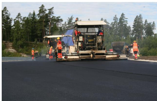
Extensive laboratory tests and trial sections were not performed due to tight time constraints. A tailored mix design was crucial, however, to get the required properties. Based on experience, Nynas Endura F1 was chosen as the binder for the surface course. The pavement of the race track will not be subjected to heavy loads from trucks, for instance; but fast cars at high speeds require good skidding resistance and cause high lateral stresses within the material they are running on.
