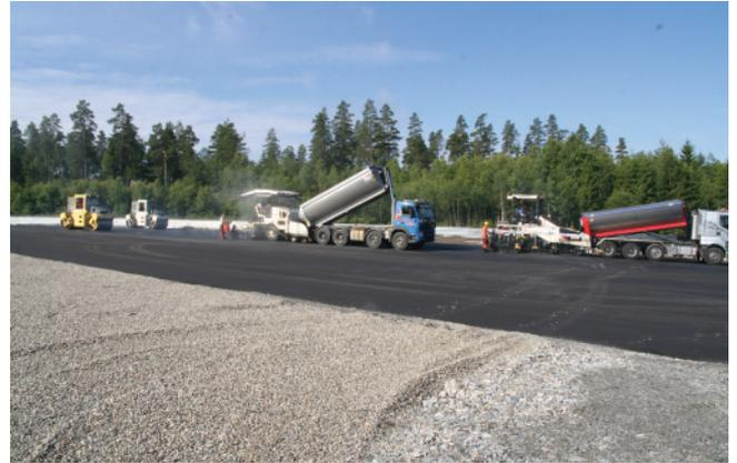
evenness were critical criteria as far as the client was concerned. The contractor Veidekke Industri was allowed to have just two joints around the 3.3km long track, both of their locations being pre specified. In the event, Veidekke Industri was praised for the evenness of track surface.
